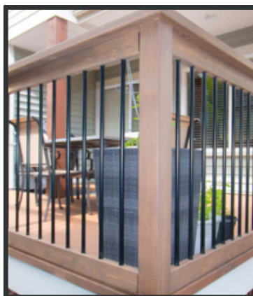
Railings PT + Aluminum Baluster
